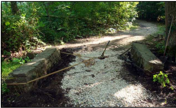
Repositioning the side walls of the bridge to make it more stable.
